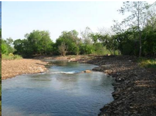
Repairs after the 2011 April Flooding
