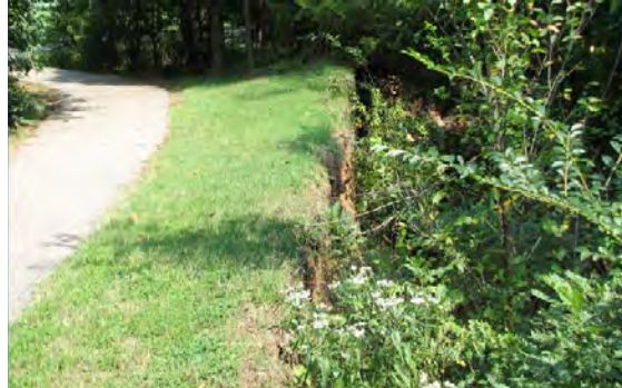
Eroded Urban Stream Bank
