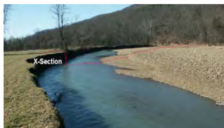
Stream bank erosion before
