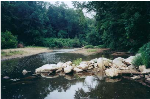
War Eagle Creek – 1 year after construction (notice formation of gravel between weirs)
