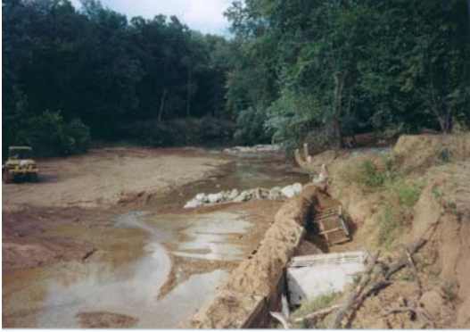
War Eagle Creek – Bendway Weir with Gabions
